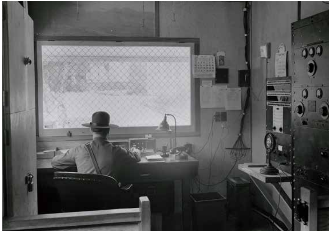
The guard control room at Tuna Canyon Detention Station
