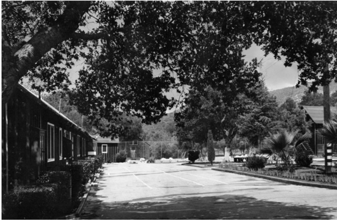
Recreation building on the left, infirmary in the distance, barracks on the right.
